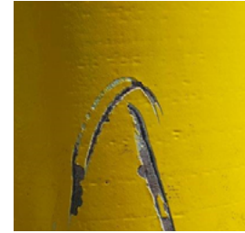
Remedial Coating Repairs Southern North Sea, UK
