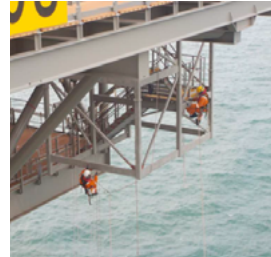
Rampion OSP Completion Phase Newhaven
