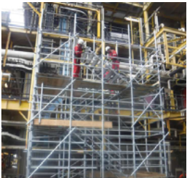
PC Platform Staircases Sole Pit Clipper SNS
