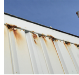
Remedial Coating Repair Project North West, UK
