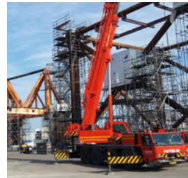
Engineering success factor in building Allseas test frame Vlissingen, NL
